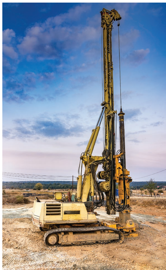
Piling rig boring foundations for tower legs
