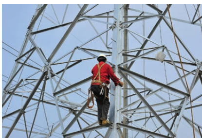
Steel tower sections
